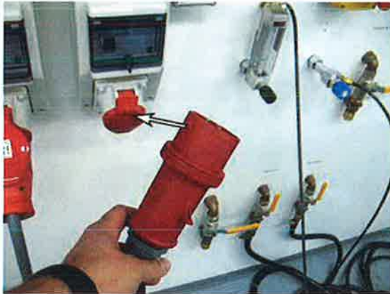
Figure 8.6: Reconnect to the mains power
